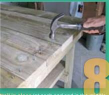
Nail in place (at each end and in the middle of the table), then tidy the edges with sandpaper. Paint or stain – or leave au naturel.
