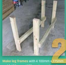
Make leg frames with 4 100mm x 775mm and 2 100mm x 1075mm (crosspieces). Screw latter 250mm up from bottom.
