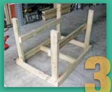
Attach leg frames to benchtop frame. Drill pilot holes and screw, using 2 screws per leg. Leg frames sit inside benchtop frame.
