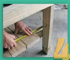
**Turn frame upright**. Lay 6 lengths 150mm x 740mm on the frame to make a shelf. Measure the gap and cut 7th piece to fit.
