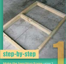
Make the benchtop frame using 2 100mm x 1150mm pieces and 3 100m x 740mm. Drill pilot holes and screw together.
